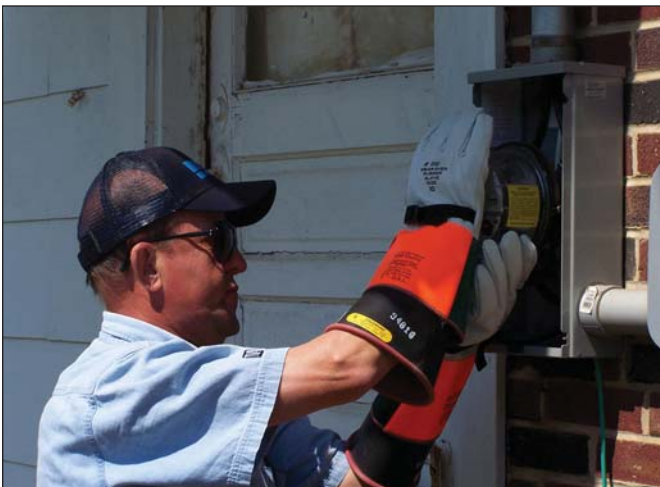
Morris Carothers installs a turtle meter. Once a turtle meter is installed, it transmits a reading back to the office every day.
