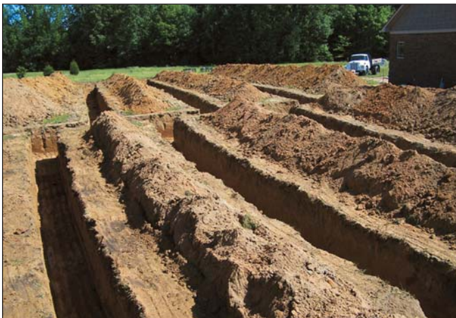
Trenching will make this system more expensive up front than traditional heating and cooling systems, but the energy savings will offset the cost in about five to six years.
